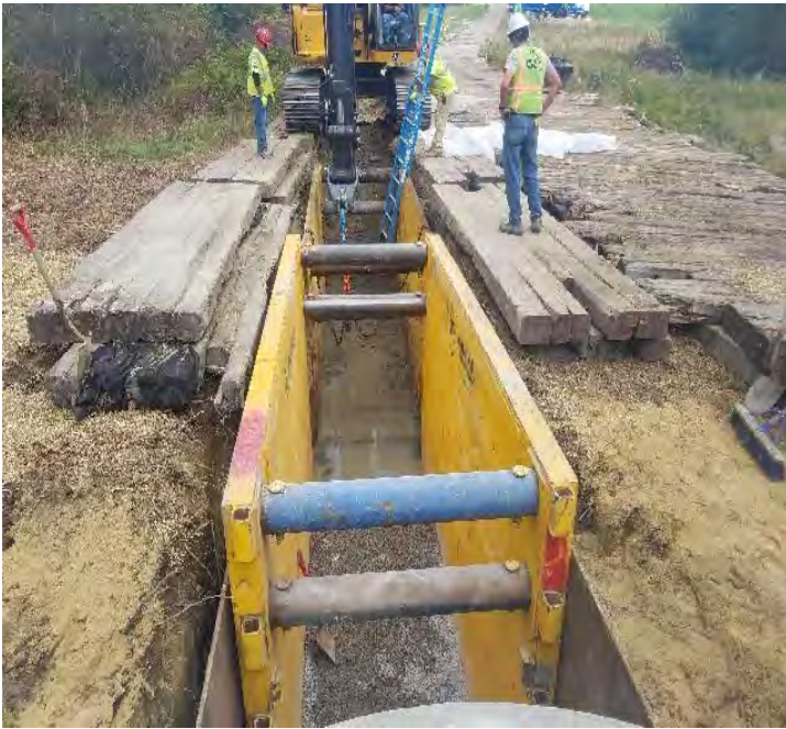
Fig 9: Trenching at Str. 106 at the Frink farm. Viewing northeast. (9-30-19).
