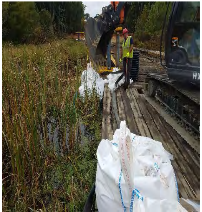
Fig 16: Commencing install of stream diversion at Knights Brook. Viewing west. (10-01-19).
