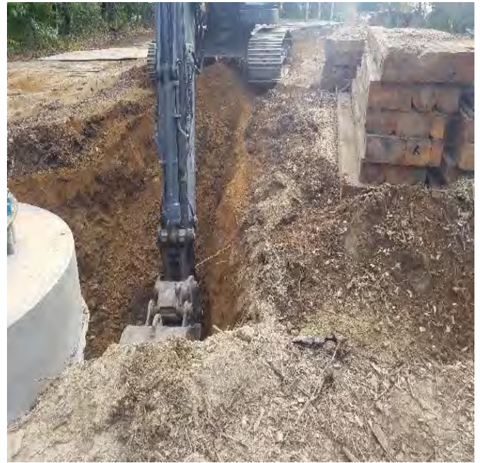
Fig 10: McCourt commencing trenching at Str. 107. Viewing southwest. (9-30-19).
