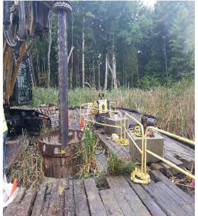
Fig 28: MJ drilling Str. 116. Viewing west. (10-02-19).
