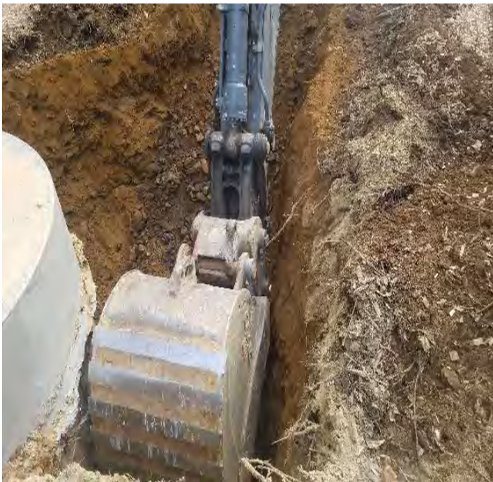
Fig 11: Trenching at Str. 107. Viewing southwest. (9-30-19).
