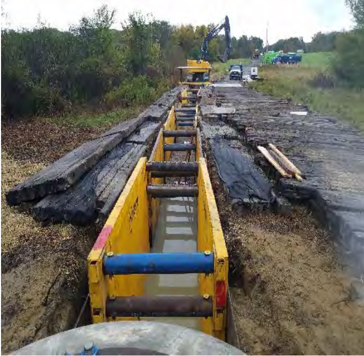
Fig 25: Continuing to trench from Str. 106. Viewing east. (10-02-19).
