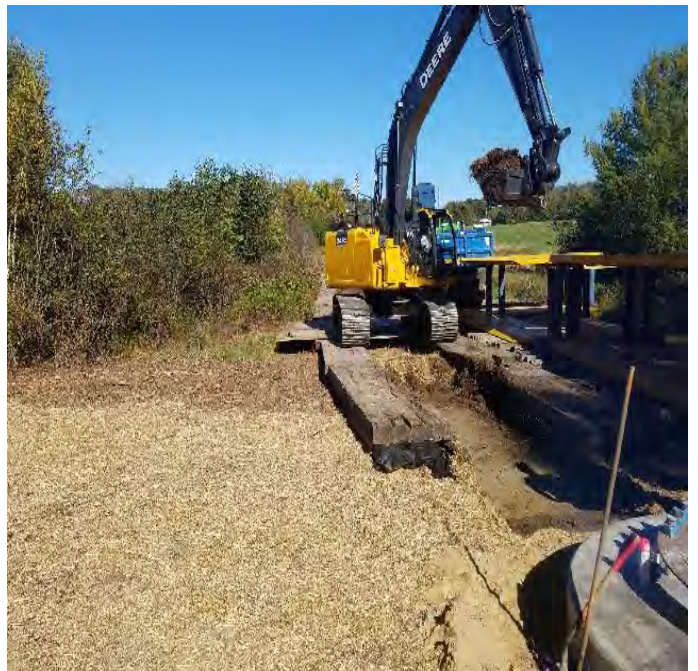
Fig 4: McCourt commencing topsoil removal at the Frink farm, starting at Str. 106. Viewing east. (9-27-19).
