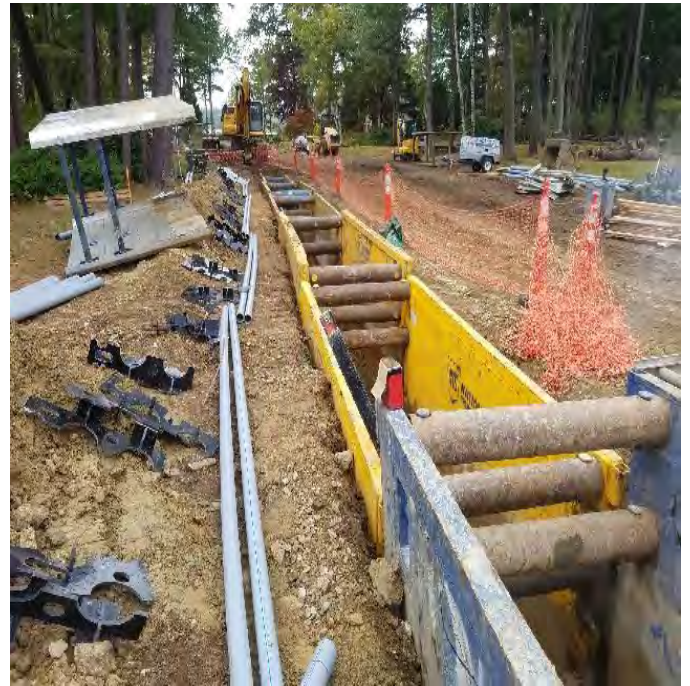
Fig 20: Trenching at the Beswick property. Viewing west. (10-01-19).
