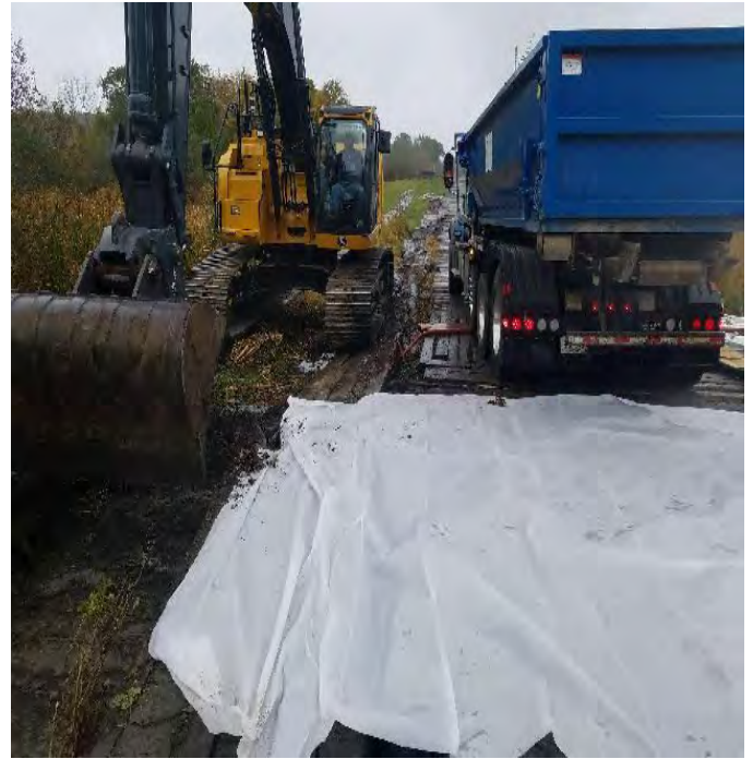
Fig 26: Prepping to remove topsoil through Knights Brook. Viewing east. (10-02-19).
