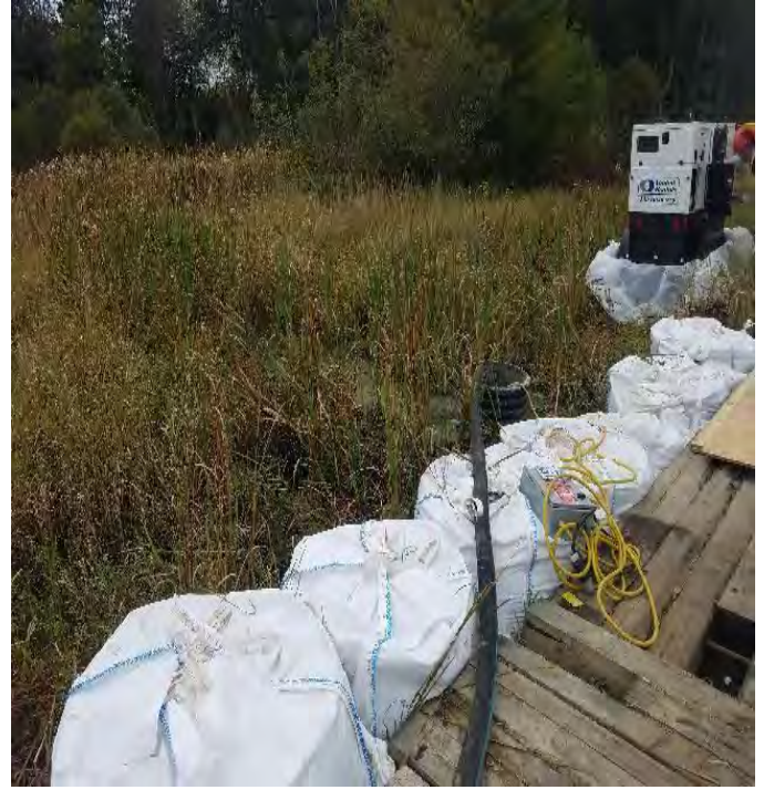
Fig 18: Stream diversion at Knights Brook. Viewing west. (10-01-19).
