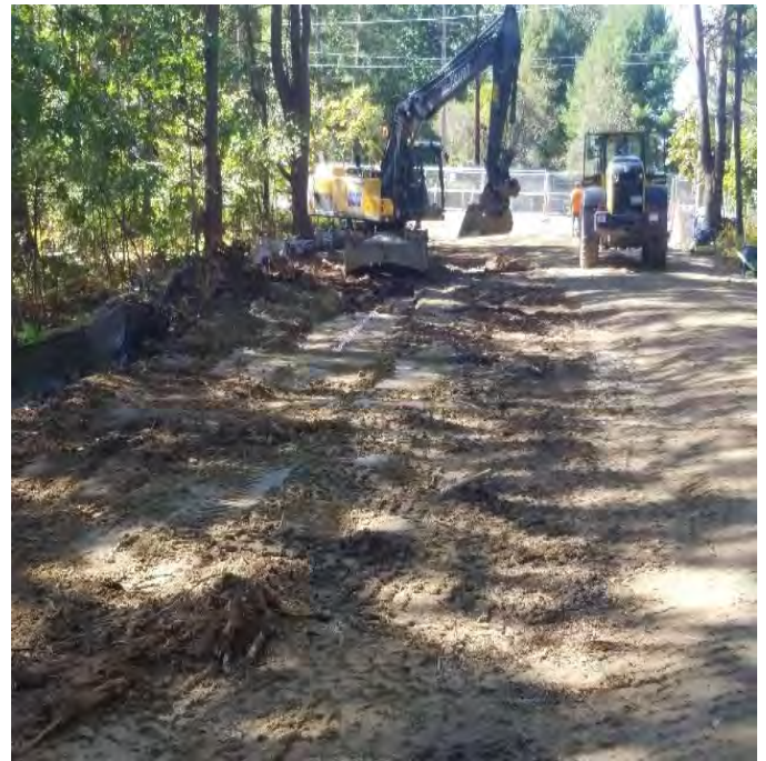
Fig 6: Backfilling trench at Flynn pit. Viewing southwest. (9-27-19).
