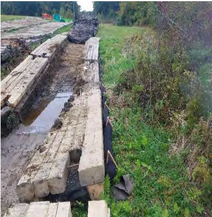
Fig 23: Filter sock installed downslope of wetland NW18. Viewing west. (10-02-19).
