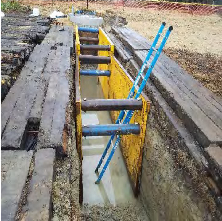
Fig 15: Overnight accumulation of groundwater in trench at Str. 106. Viewing west. (10-01-19).
