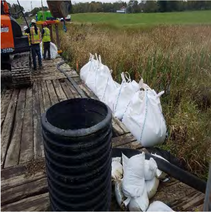
Fig 17: Installing the stream diversion at Knights Brook. Viewing east. (10-01-19).
