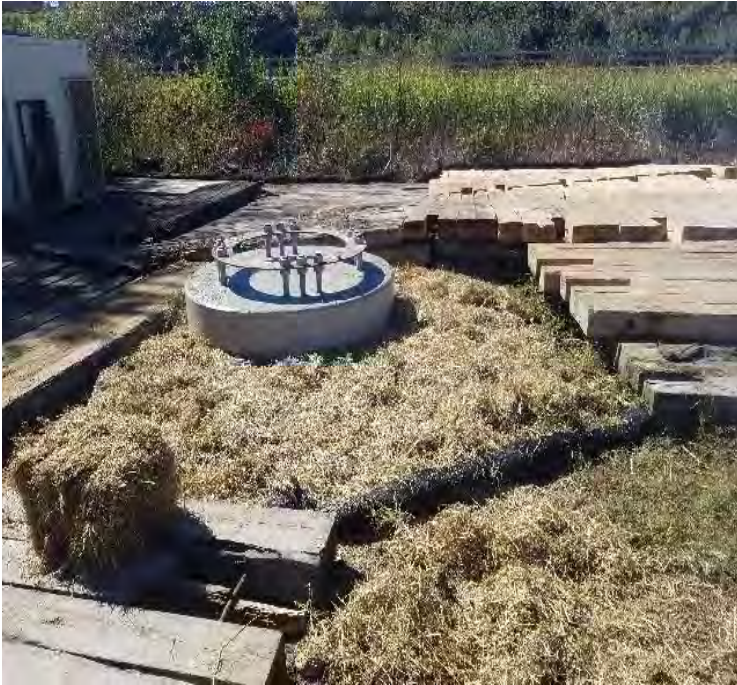
Fig 5: Str. 131 foundation. Viewing southwest. (9-27-19).
