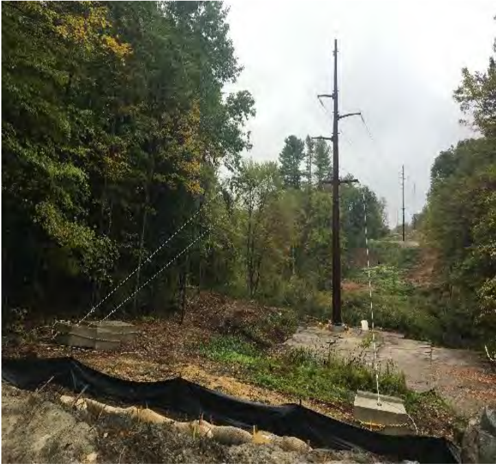
Fig 13: Str. 28 and surrounding sediment controls. Viewing north. (10-01-19).
