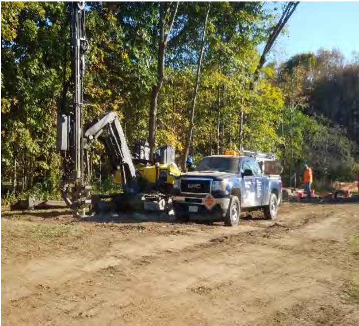
Fig 7: Maine Drilling and Blasting prepping to blast. Viewing northeast. (9-30-19).
