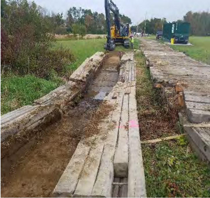
Fig 21: Stripping topsoil through wetland NW18 at the Frink farm. Viewing east. (10-01-19).
