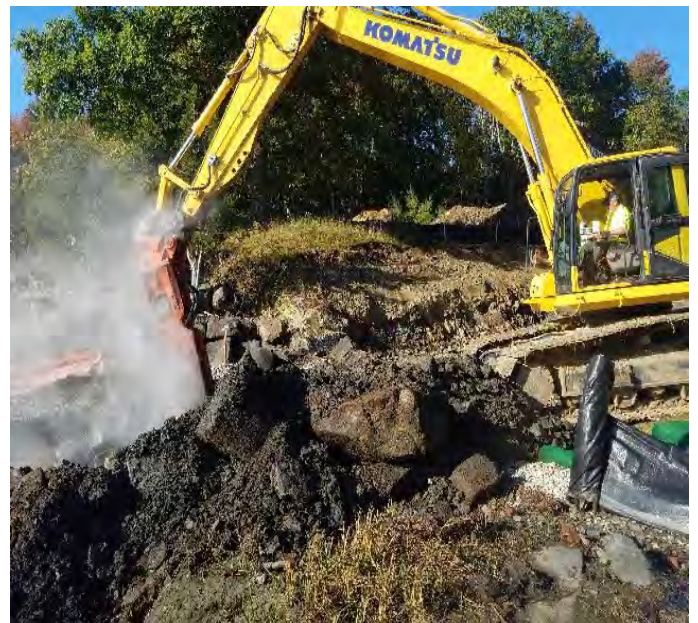
Fig 2: Blu Rock hammering ledge on Durham side of the Bay. Viewing west. (9-27-19).
