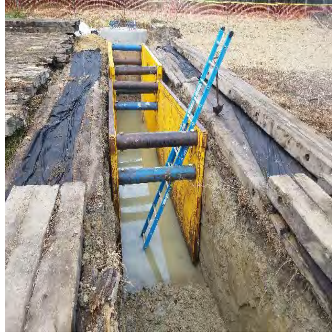
Fig 22: Overnight accumulation of groundwater in trench at Str. 106. Viewing west. (10-02-19).
