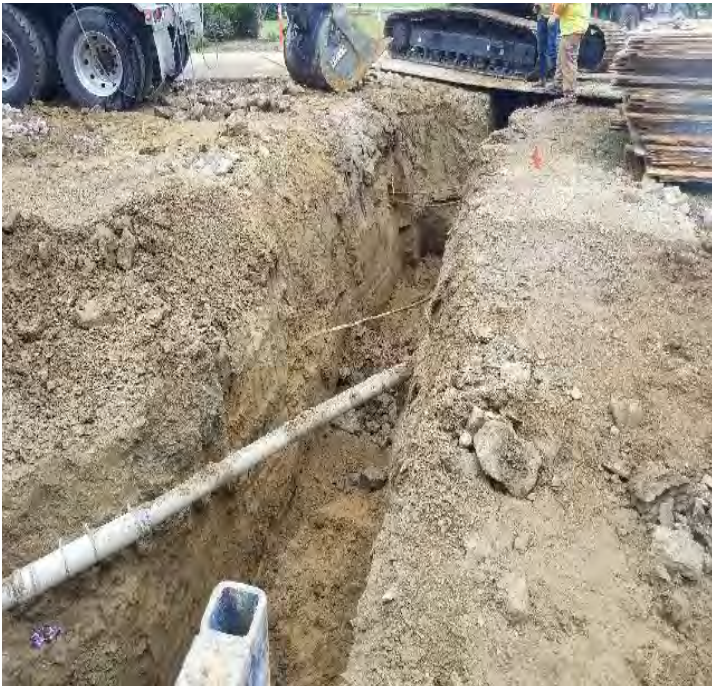
Fig 19: Excavating around exposed underground cables and pipes. Beswick property. Viewing east. (10-01-19).
