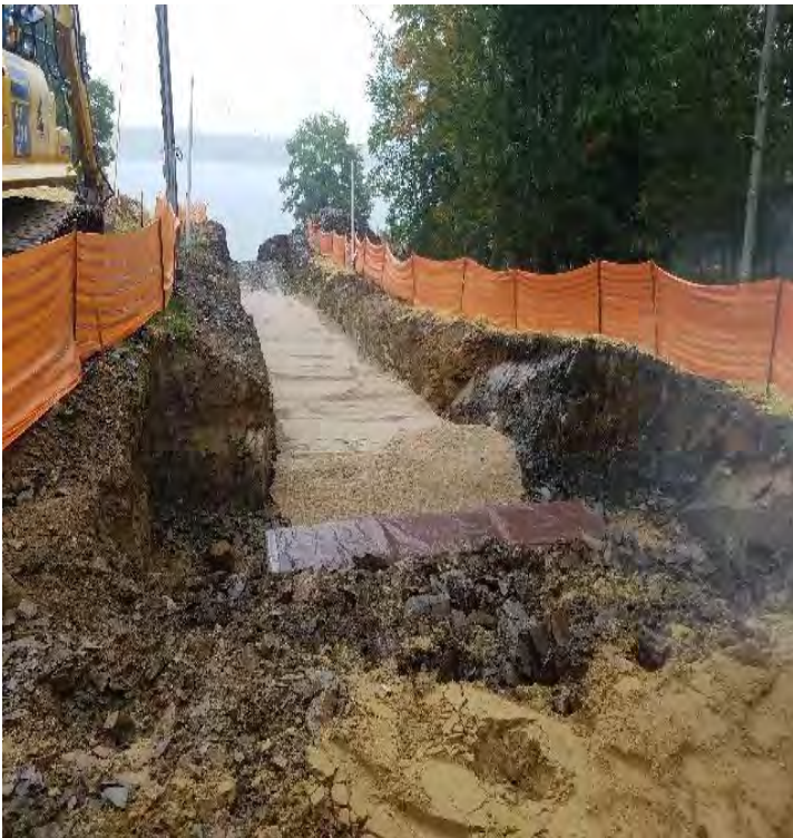
Fig 27: 6-8in of sand in trench at the cable house. Viewing east. (10-02-19).
